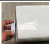
6. Retighten the **threaded ring** at the bottom of the cistern, ensuring the rubber seal remains in the correct order.
