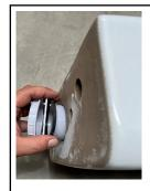
1. Unscrew the threaded ring underneath the cistern until it is completely loose.
