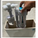
3. Remove the cistern mechanism entirely from the cistern.
